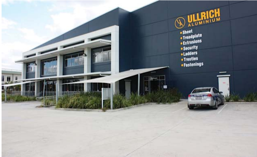
Carole Park Office, Queensland, Australia
