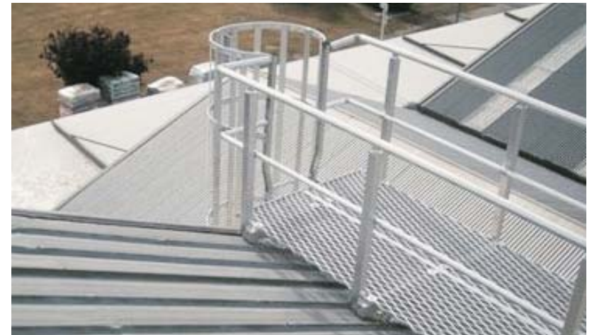
Aluminium Roof Access and Roof Walkway
