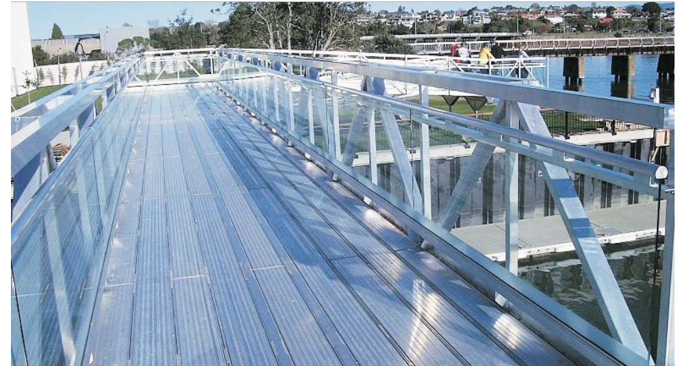
Ullrich Aluminium fabricated walkway
