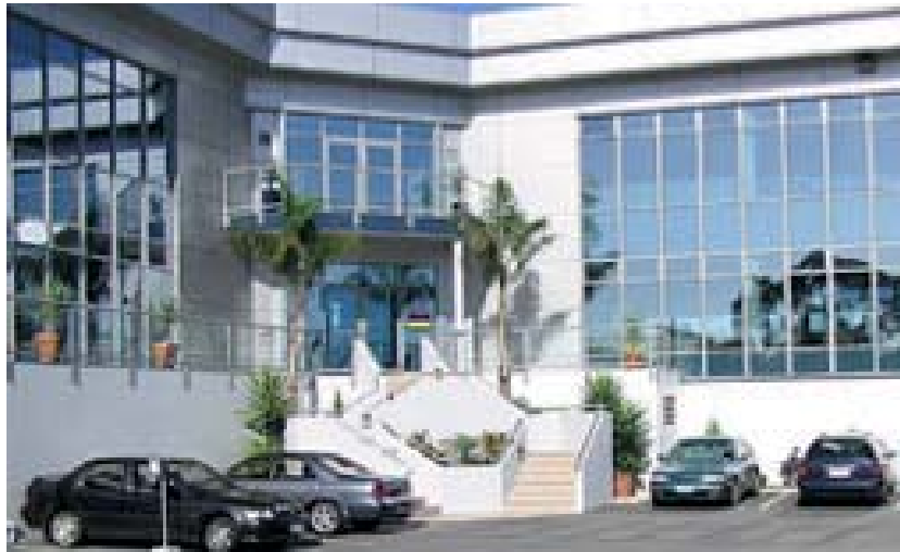
Manukau Office, Auckland, New Zealand
